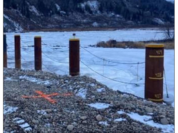
4 - Temporary Moberly River Debris Piles (example of piles)
