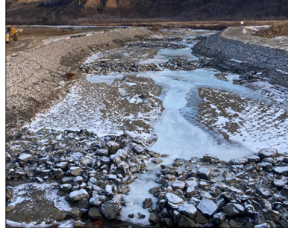
2 - Temporary Diversion at Cache Creek (similar diversion at Farrell Creek)
