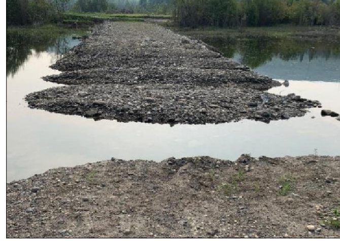
1 - Temporary Causeway for Reservoir Clearing (causeway example)
